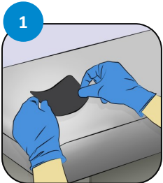
Position over damaged area.
